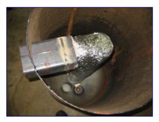
The above image shows the combustion chamber and chimney being welded into the side of the hot water tank. Note the block of wood between the end of the chimney and the inside surface of the tank to ensure an appropriate gap for the exhaust gases. This piece of wood will be removed after the chimney is welded in place.
