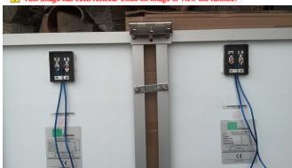
I had to wire them in parallel so I drilled out a hole in the frame to run the wires from one panel to another
