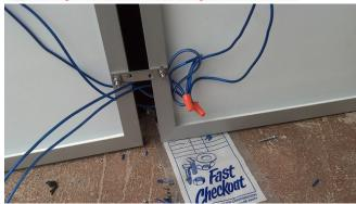
I decided to hard wire the 12 volt terminal to the battery since the inverter already clamps to the posts, so I cut off the clamps
