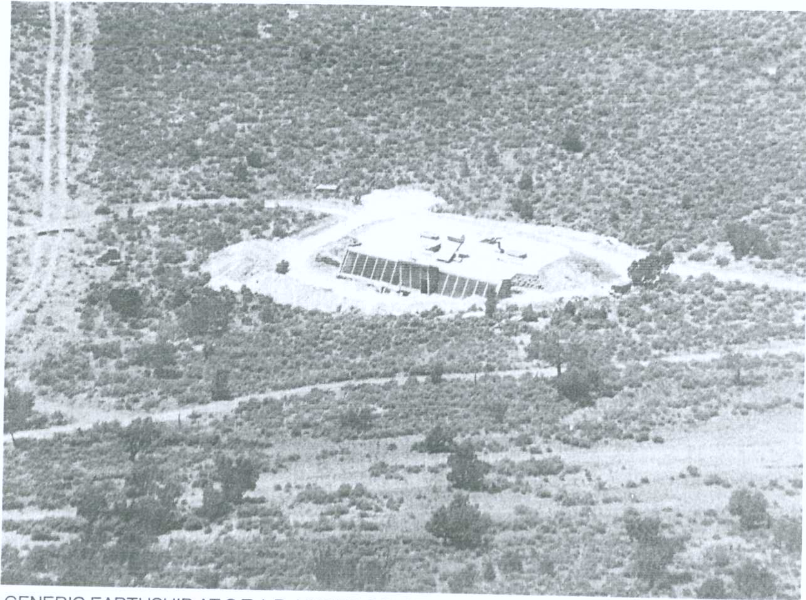
GENERIC EARTHSHIP AT S.T.A.R. UNDER CONSTRUCTION
