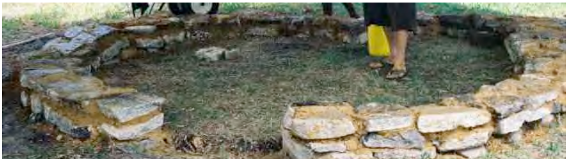
Fig. 23. Stem wall: Above ground
