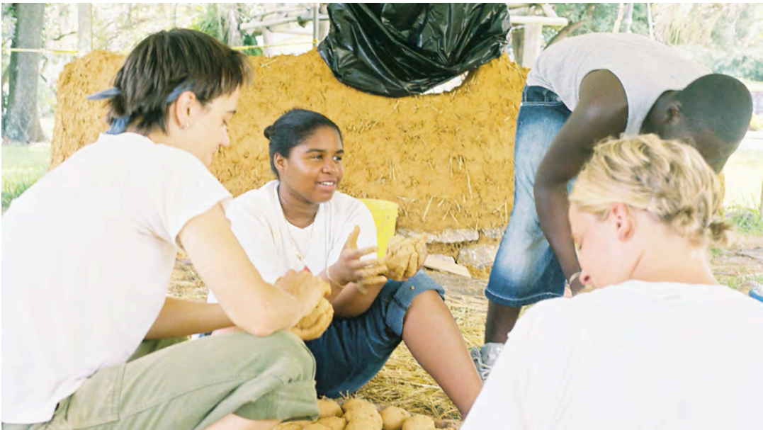
Fig. 25. Making cob balls
