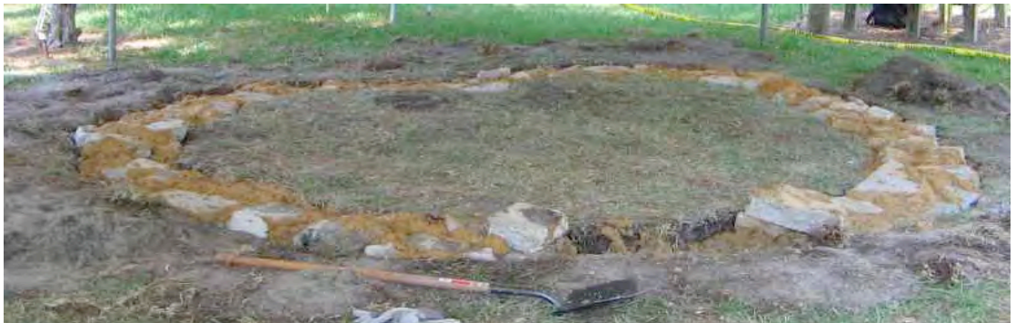
Fig. 22. Plinth wall: In the ground
