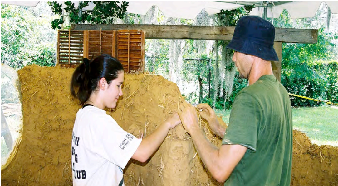
Fig. 24. Applying cob
