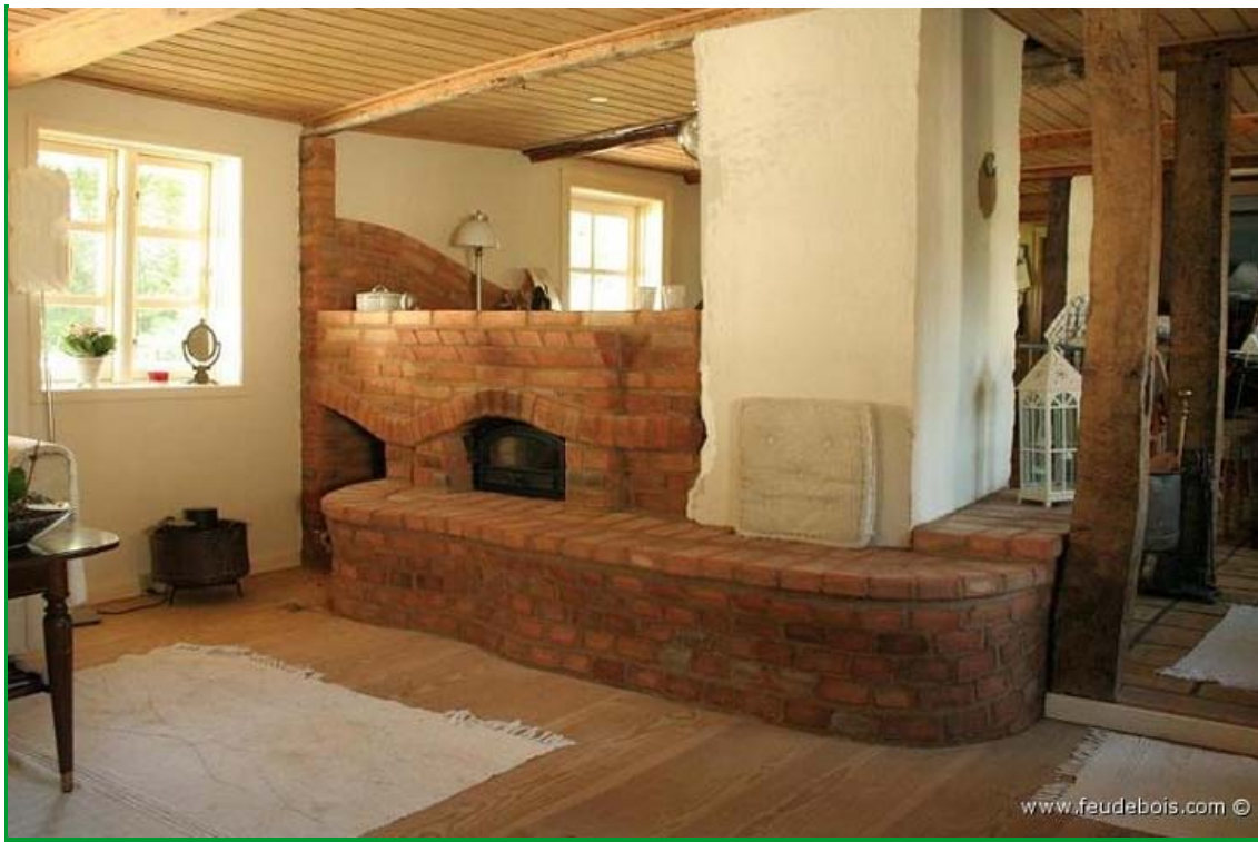
Brick masonry heater. There is no reason why some heaters can't be low and long. There is a wood fired cookstove on the opposite side of this heater. stenovne.dk
