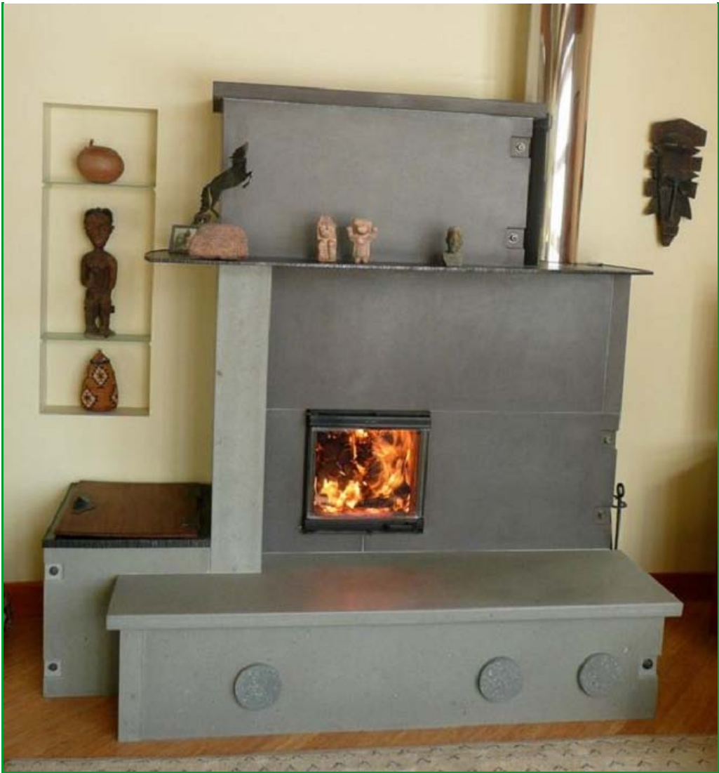
Masonry heater that extends to room on other side of wall. Custom concrete slabs, steel, black walnut wood box top, bluestone, lilac bluestone. By turtlerockheat.com
