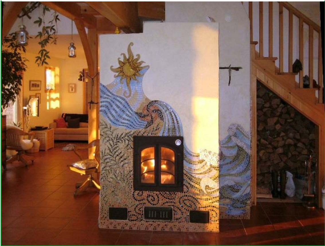
Stucco and mosaic masonry heater. Core is by Heat-kit. www.mha-net.org
