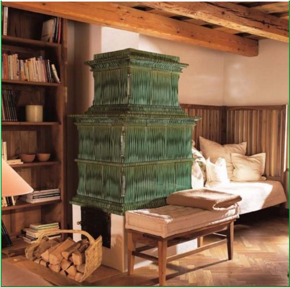
Tiled masonry heater with Asian influence. Only special 'kachel' tiles can touch the inner firebrick, all other tiles must be spaced away from the inner masonry, otherwise they will crack. fliesen-ofen-ritter.at
