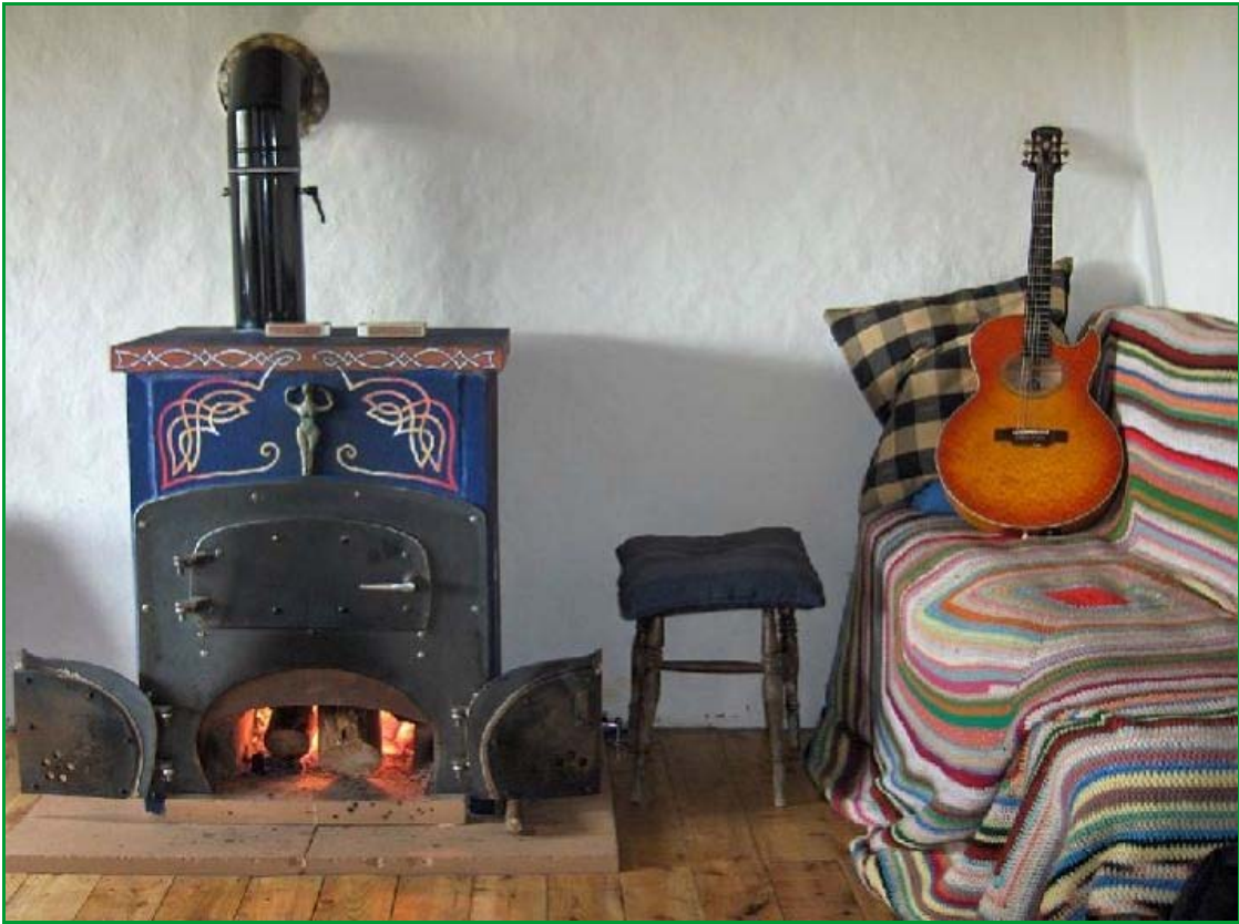
A masonry heater made from paving slabs. But, this heater most likely will not pass
