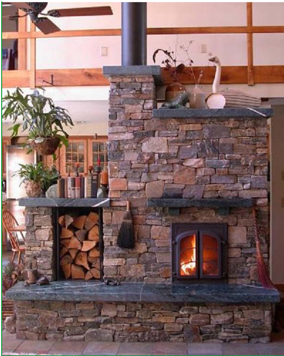
This masonry heater in Burlington, Vermont has a bake oven on the kitchen side. Masons: William Davenport, Spencer Blackwell, Norbert Senf. turtlerockheat.com
