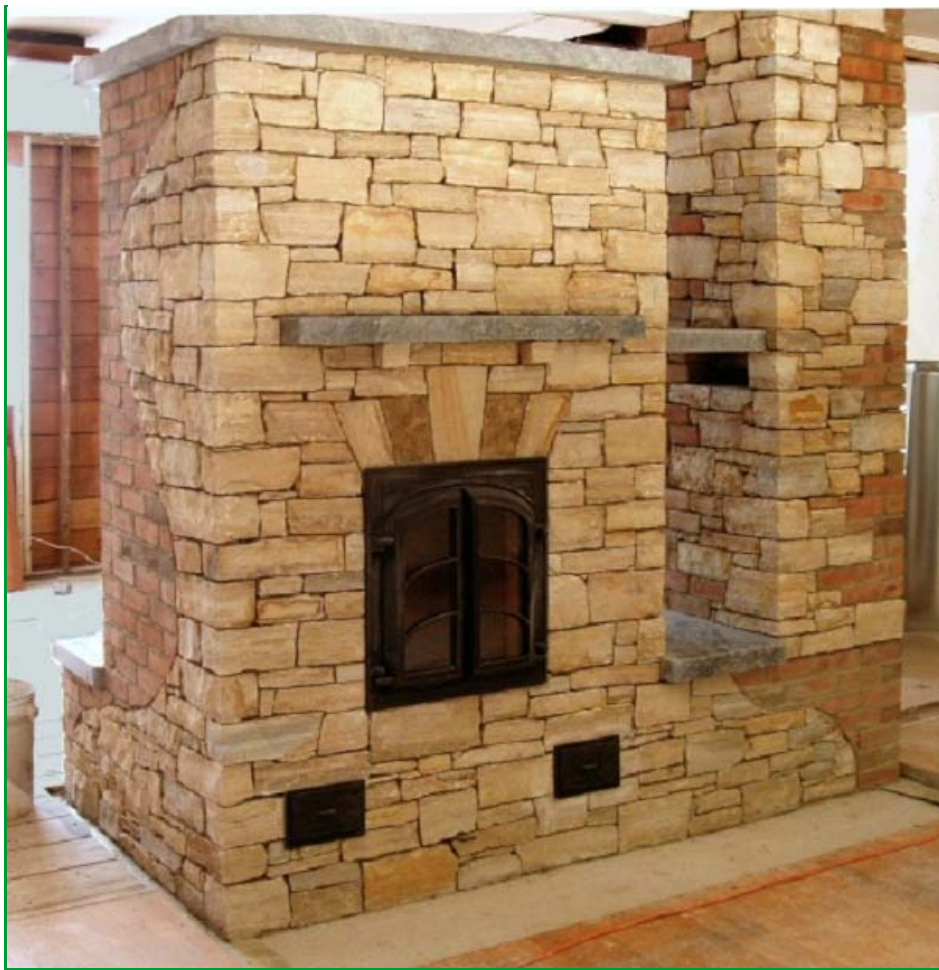
Masonry heaters are best positioned in the center of the home. The kitchen side of this heater is faced in brick. Massachusetts heater by Steve Bushway, ultimateridgehook.com . Core by heatkit.com
