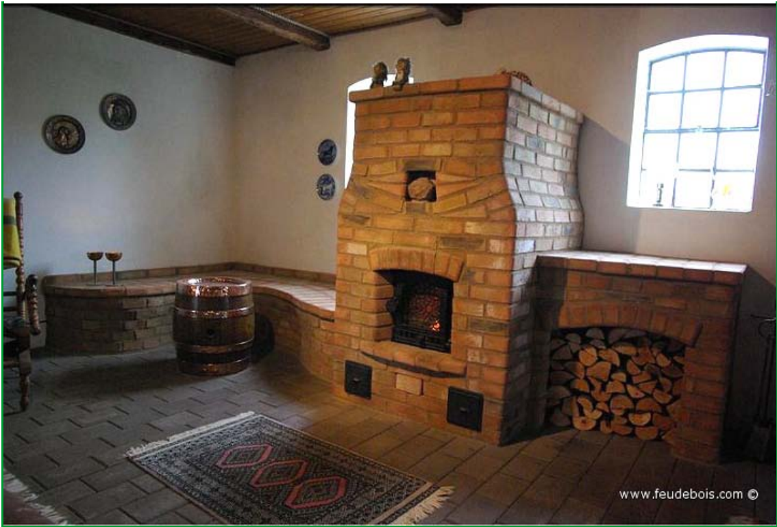
Brick masonry heater with heated bench in France by feudebois.com. A heater with a façade thickness of 3-4 inches, gives a moderate heat transfer, not too fast, not too slow.
