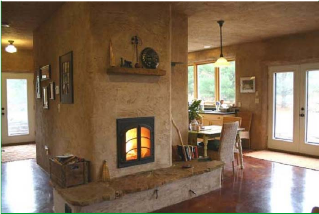
This masonry heater is veneered with the same earth-clay plaster used on the walls of the main floor. A heated bench topped with sandstone makes for a warm perch on winter days. By Gimme Shelter Construction. gimmeshelteronline.com
