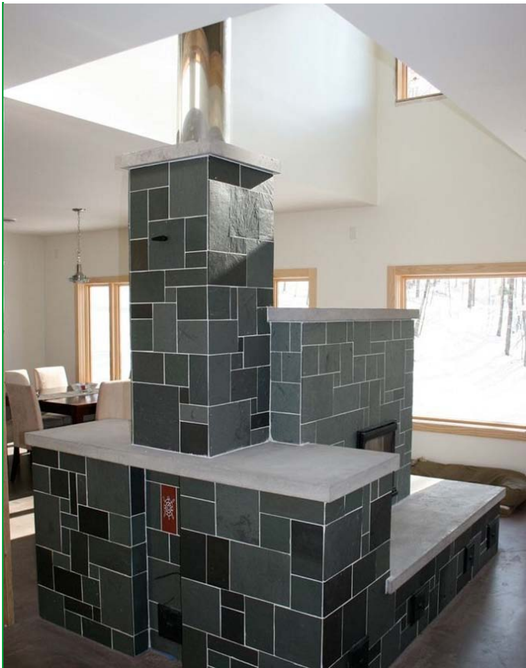
Local slate covers this masonry heater in Vermont by William Davenport. The heater has doors on both sides. turtlerockheat.com
