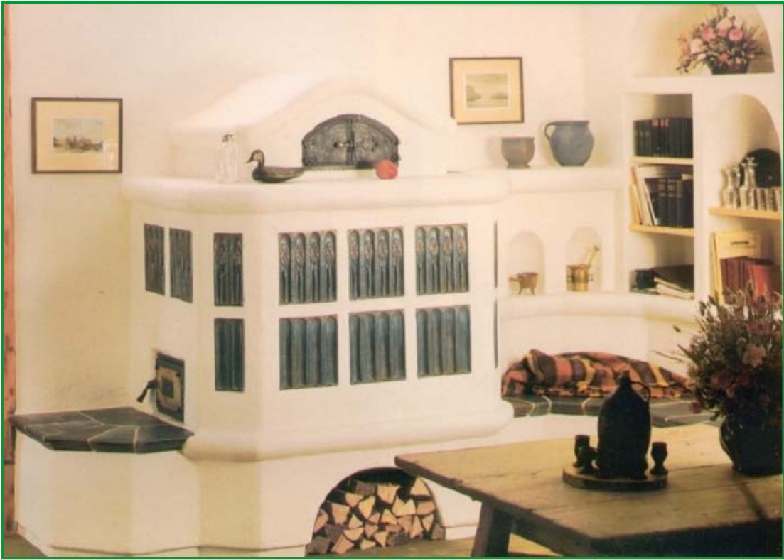
Tiled masonry heater with Asian influence. Only special 'kachel' tiles can touch the inner firebrick, all other tiles must be spaced away from the inner masonry, otherwise they will crack. fliesen-ofen-ritter.at
