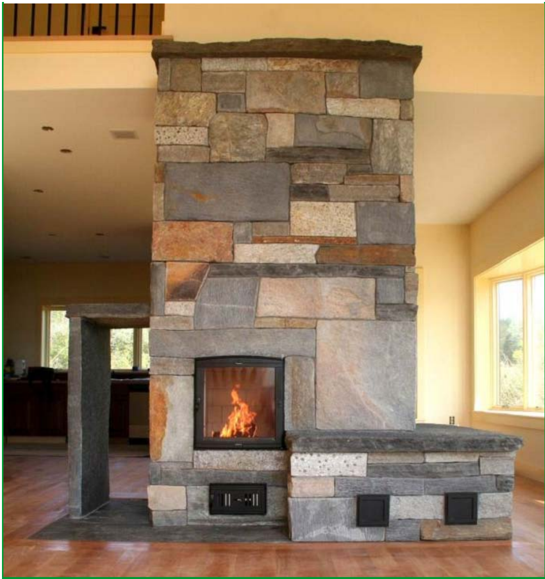
Masonry Heater with wrap around heated bench, direct fire oven (on kitchen side), and wood storage by Carsten Homstead of Massachusetts. homespunworks.com
