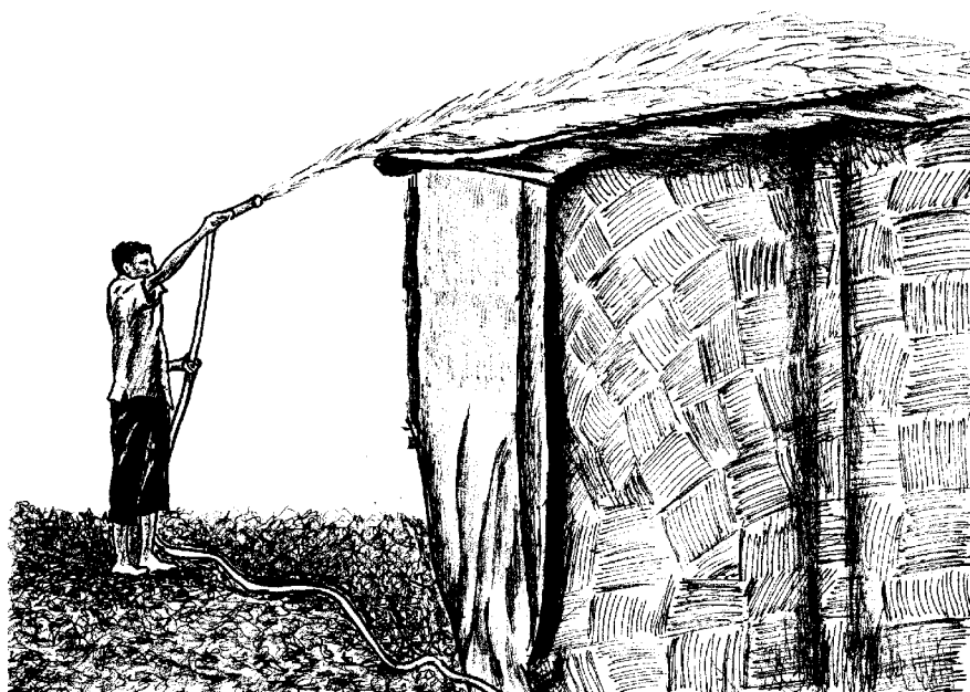
Figure 26: Spraying the jute-covered roof
