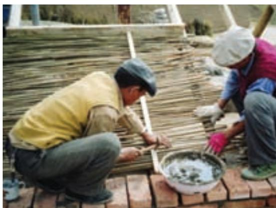
Figures 65 & 66: A roof structure made of timber and bamboo (Qinghai)
