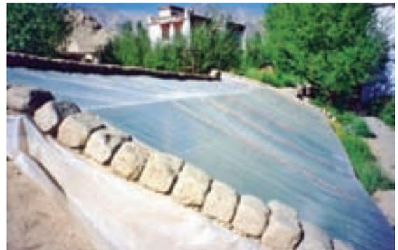
Figure 76: Close-up view of fixing the polythene sheet with mud bricks laid on a mud coating
