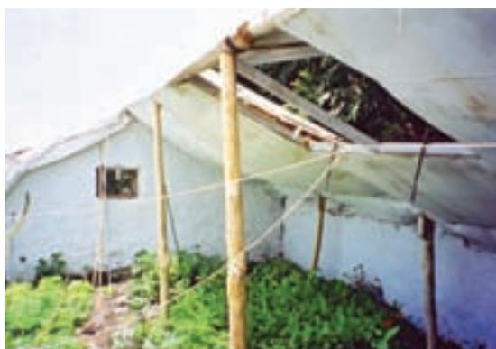
Figure 72: Open roof shutter from inside
