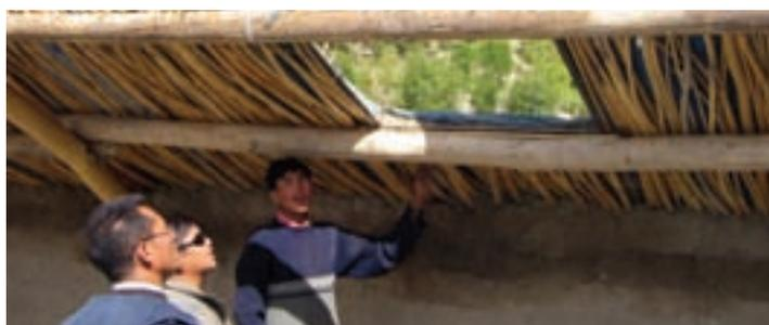
Figure 15: Opening the roof ventilator
