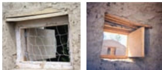
Figures 53 & 54: Inside and outside views of installed side shutter with chicken mesh outside
