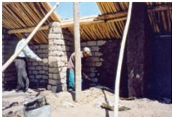
Figure 41: Finishing off the partition walls
