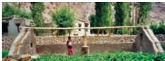
Figure 57: Roof structure with two beams and shutter frames in position in Spiti
