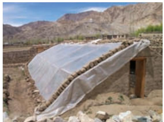
Figure 77: General view of fixing of the polythene sheet
