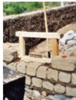
Figure 52: Positioning the shutter frame on the wall
