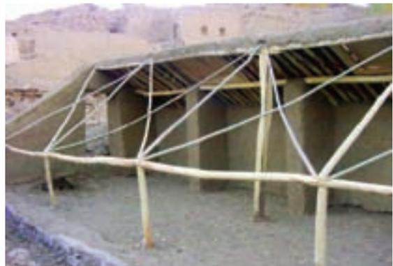
Figure 42: Completed inner partition walls, greenhouse in Zeback district, Afghanistan
