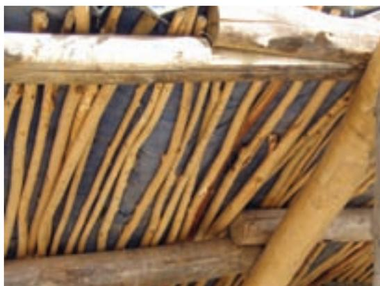
Figure 61: The layer of sticks forming the underside of the roof
