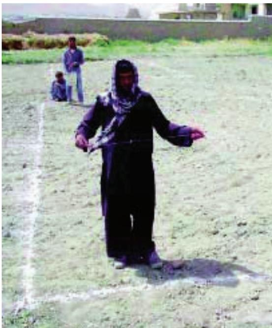
Figure 31: Marking the position of the walls
