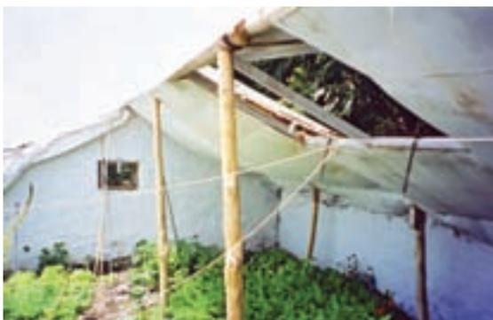
Figure 63: A white cloth added under the roof
