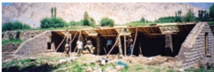
Figure 13: Greenhouse under construction (view of the double walls and the structure of the roof)
