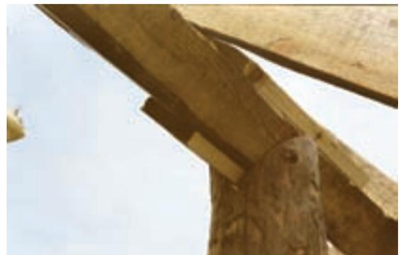
Figures 56: Fixing the beam to a post, Ladakh (top) and Qinghai (bottom)
