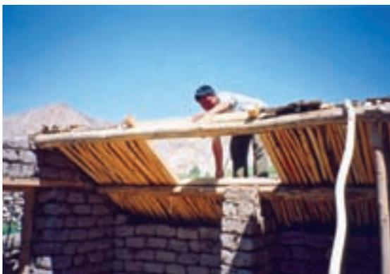
Figure 70: Fixing the frame of the roof shutter
