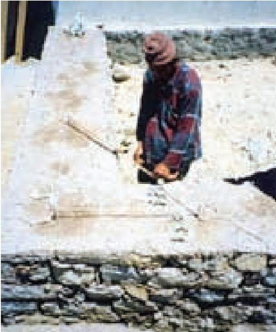
Figure 28: Drawing a right angle using the '3,4,5' method
