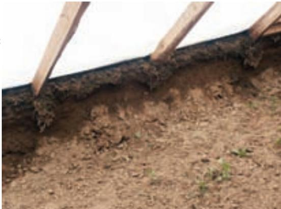
Figure 75: Joists balanced on a crumbling earth layer (outside ground level) in a greenhouse without southern foundations
