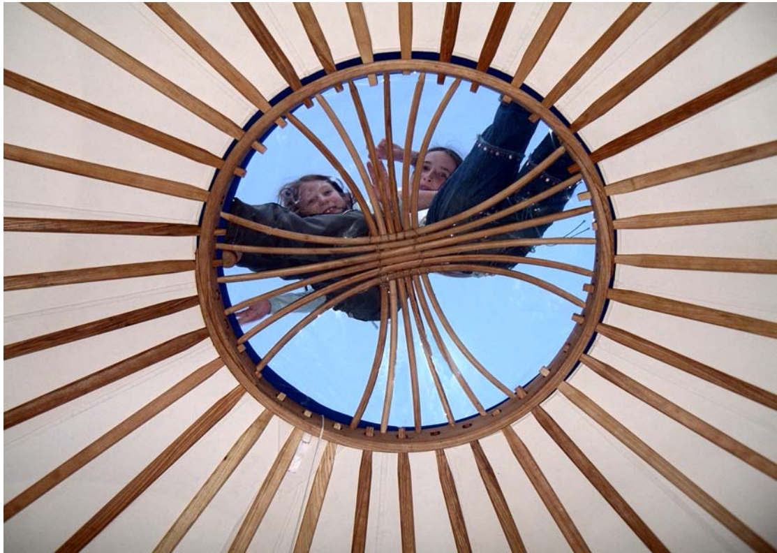
Going to extremes in yurt inspection!
