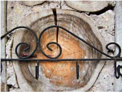
Above: As expected, some timber splitting and mud cracking has occurred – easily fixed with more mud.
