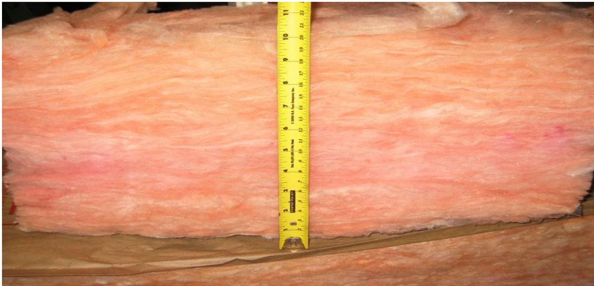
Slight update - as suggested, I extended the thickness of the walls two inches by adding a 2"x2"x8' to each joist. I also got some proper strapping which made the job go a lot quicker. I didn't take the insulation all the way out but I did re-fluff it as much as possible. There are still some small spots I need to fill, but overall - the walls are done. Here are two photos:
