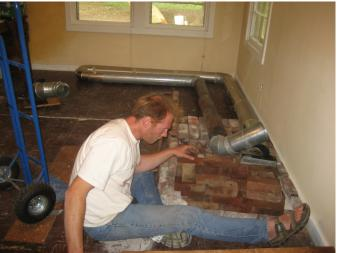
temperatures tend to stay below 600 F, so galvanized ducting can be used throughout.
