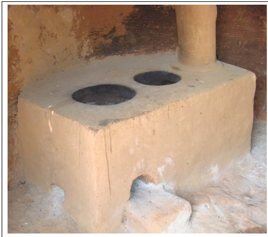
Photo 13: The Finished Rocket – Lorena Stove
