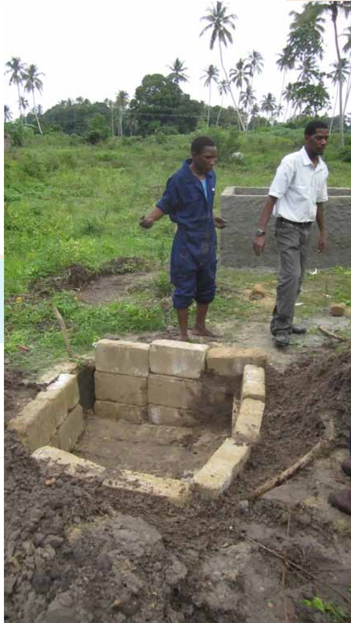
A photo showing the (1m width x 1m length and 0.7m depth) brick-lined kiln
