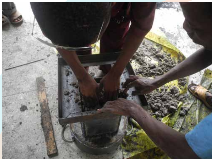
Photo showing the filling of the cavity around the 'elbow'
