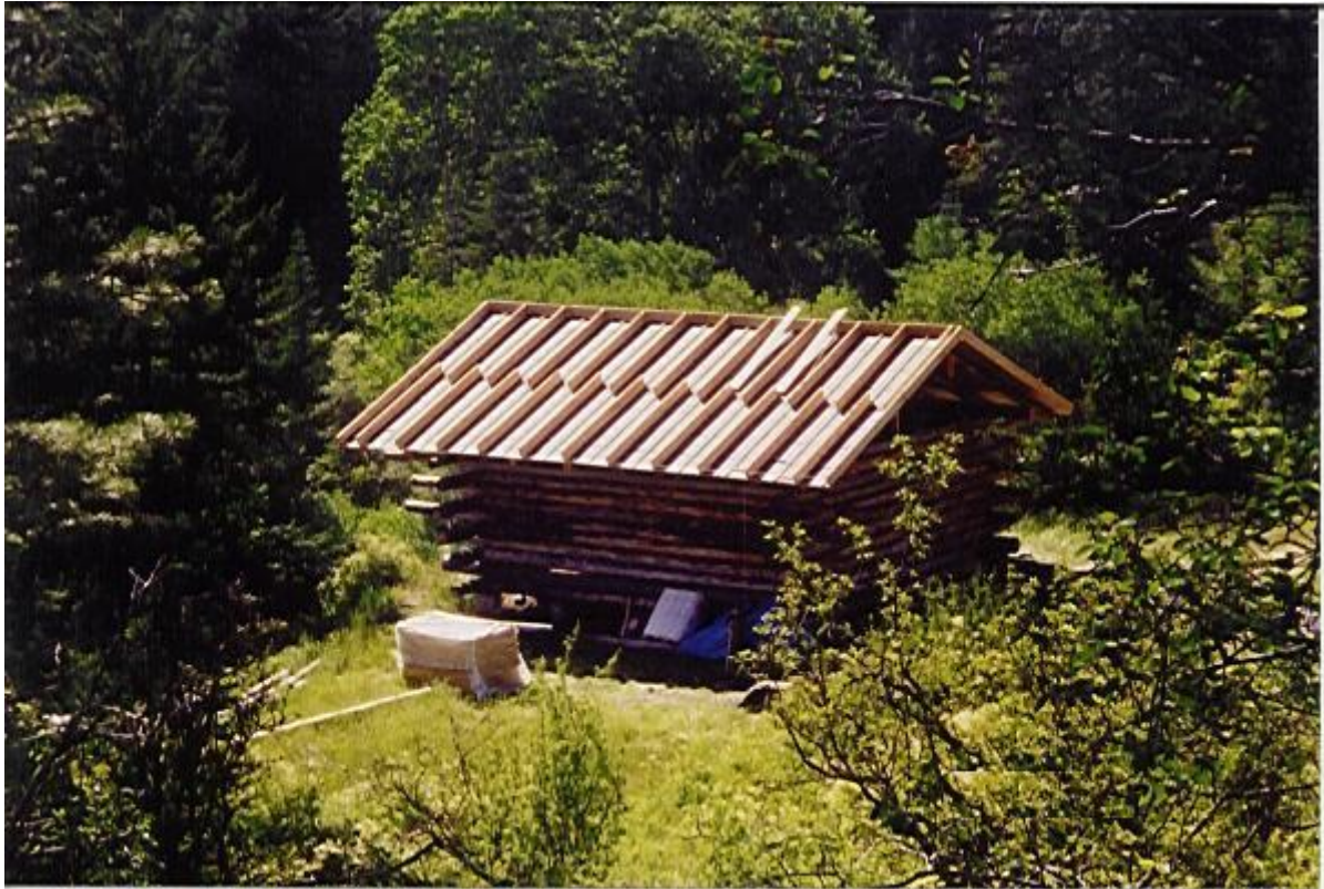
(Photo above) We added 2x10 rafters all screwed and toe nailed to the 2x2s so that we could transfer the loads down to the 2x6 fir which is our structural roof.
