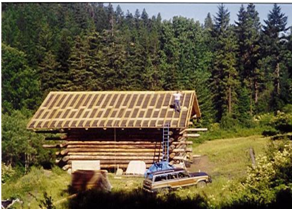
We added 2x8 blocks between the rafters to stabilize the roof. The roof was designed to ventilate from eave to peak over the top of the insulation and over the blocks
