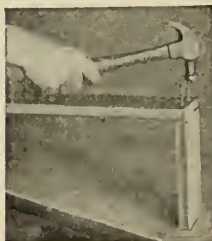
FIG. 9.—“Toe-nailing” (at right) calls for more practice.
