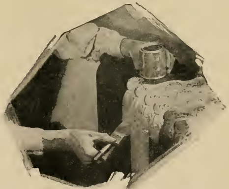
FIG. 22.—Flat-drying paint of the kind often used for walls is ideal for decorating the radiator coils.
