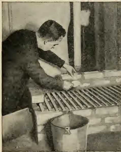
FIG. 22.—All the combustible waste of the household can be burned in this type of incinerator. At the left is shown how the brick walls are laid up after the first grate bars are in place.
