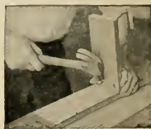
FIG. 8 (left).—Handling a hammer for straight nailing. Note that it is gripped near the end.
