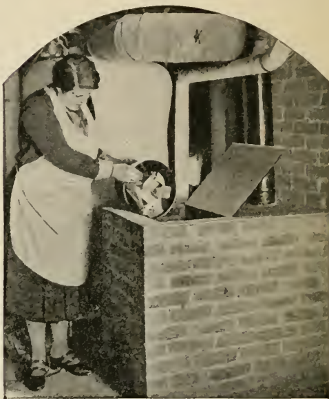
FIG. 22.—All the combustible waste of the household can be burned in this type of incinerator. At the left is shown how the brick walls are laid up after the first grate bars are in place.
