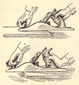
Fig. 29-Starting the Plane and Finishing "bring out" and em-
